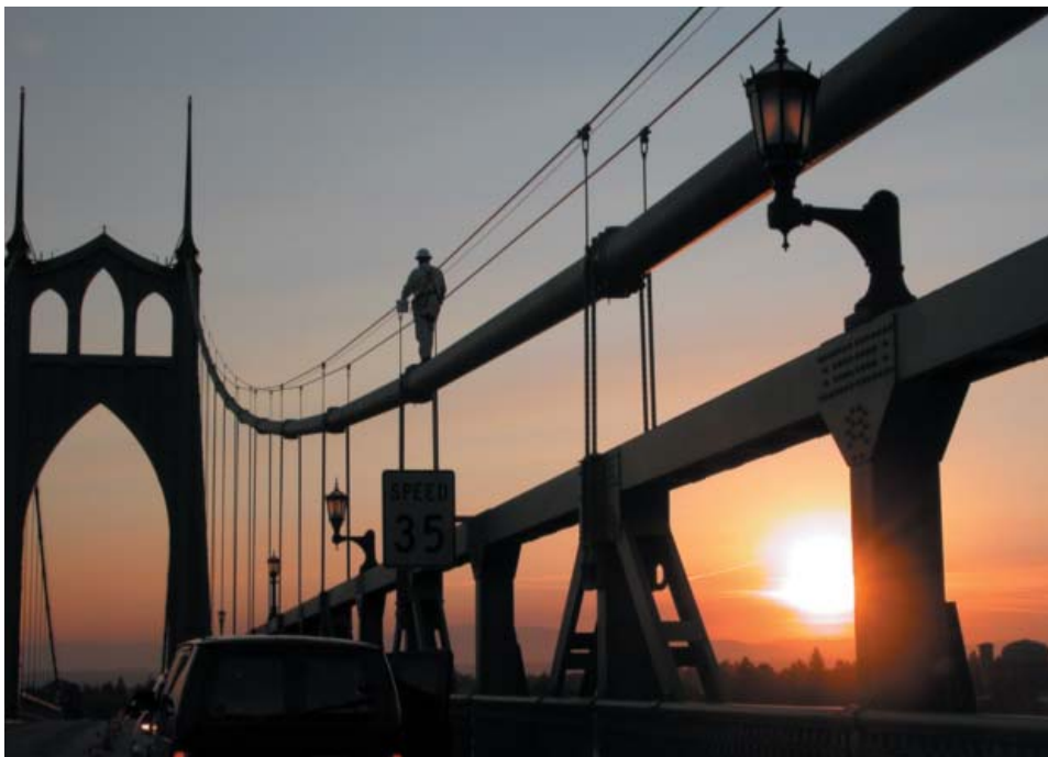
Finishing Trades journeymen painters applied their skills and modern touches to the historic St. John's Bridge in Portland.
