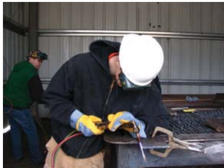
Welding at the Ironworkers.
