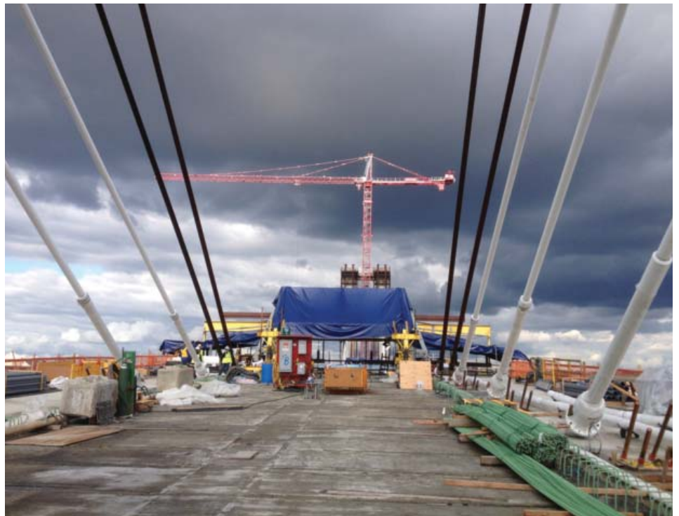
Willamette River Bridge, courtesy of Tyler Street.
