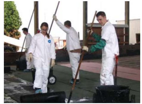
Laying tar at the Roofers.
